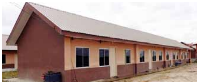
Worker's quarters at Miri estate
