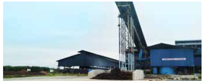
PTNJL's composting plant
