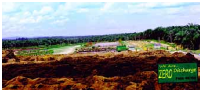
Composting, ETP and POME application at PTNJL
