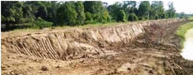
Construction of bunds at Miri estate
